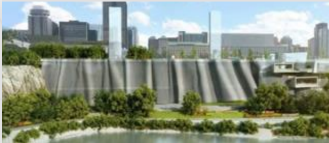
Cliff Energy Centre
