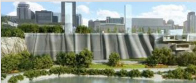
Cliff Energy Centre
