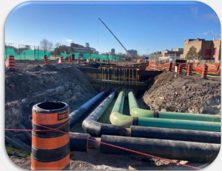
Underground Distribution (Piping) Network Construction 2022
