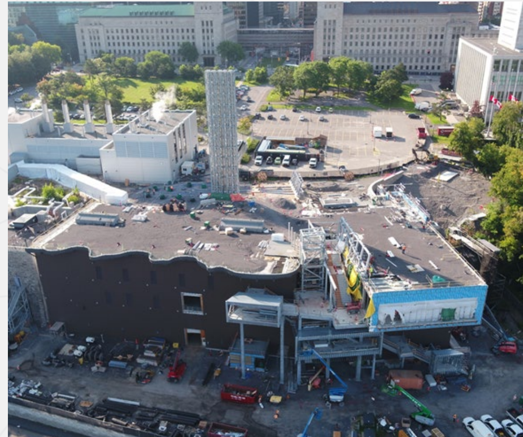
Cliff Energy Centre Construction – August 2023
