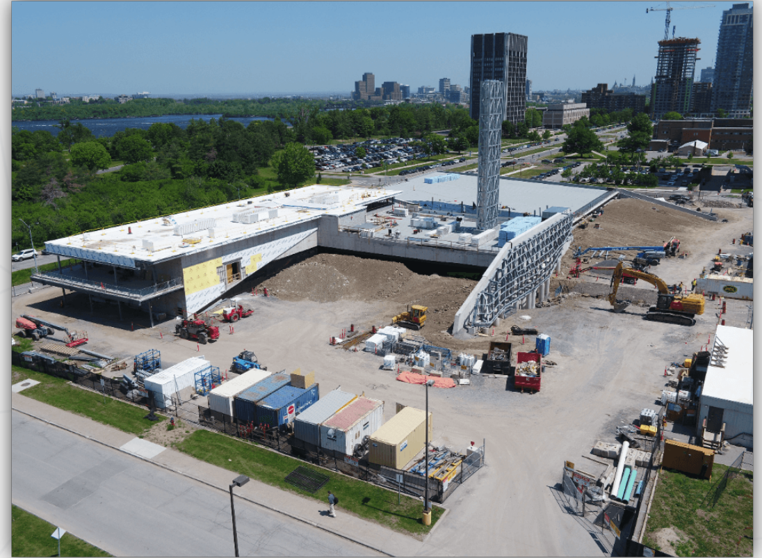
Tunney's Pasture Construction – May 2023
