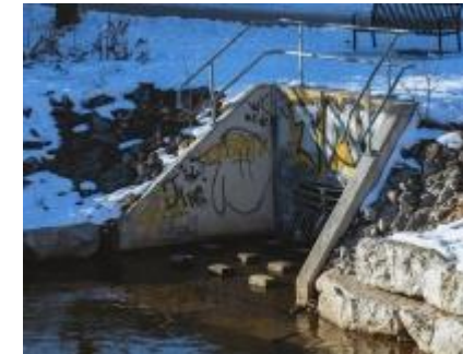
Storm and sewer
