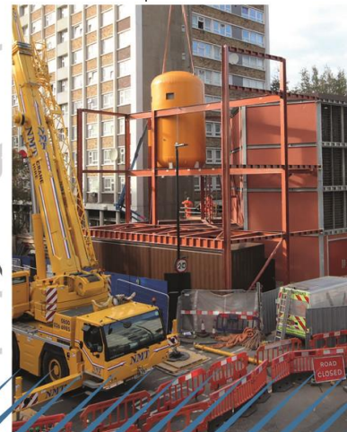
Boiler craned into position
