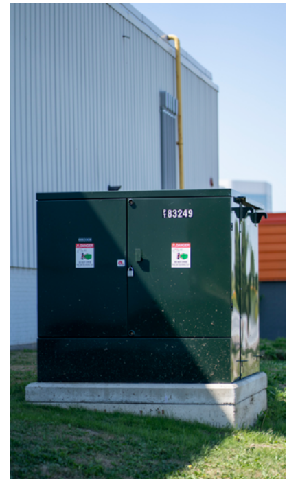
FIGURE 8: Pad-mounted transformer ■ Customer’s responsibility ■ Toronto Hydro’s responsibility
