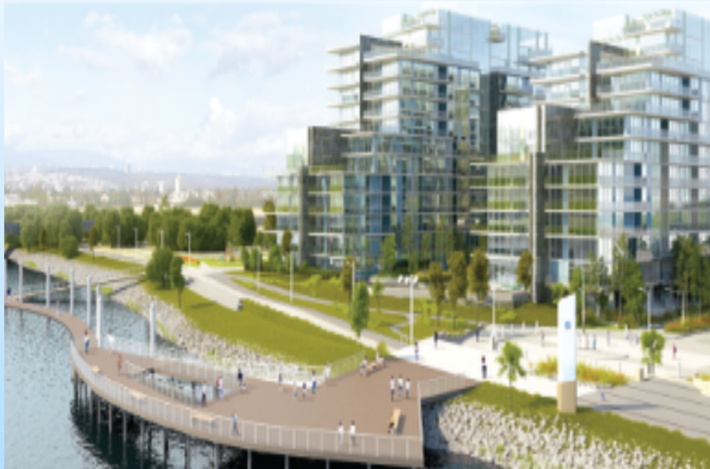
Geothermal at Lulu Island in downtown Richmond, BC, expansion will take it to 50 M sq ft, cutting GHG 34,000 tonnes per year.
