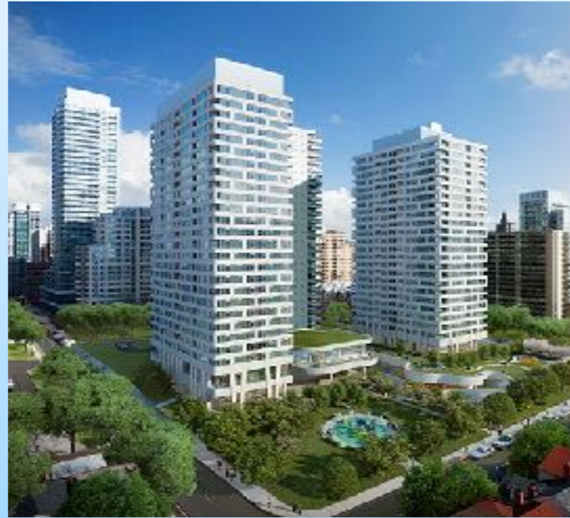
TORONTO CONDOS AT LILLIAN PARK GEOTHERMAL SHARED WITH CITY SENIORS TOWER NEIGHBOUR
