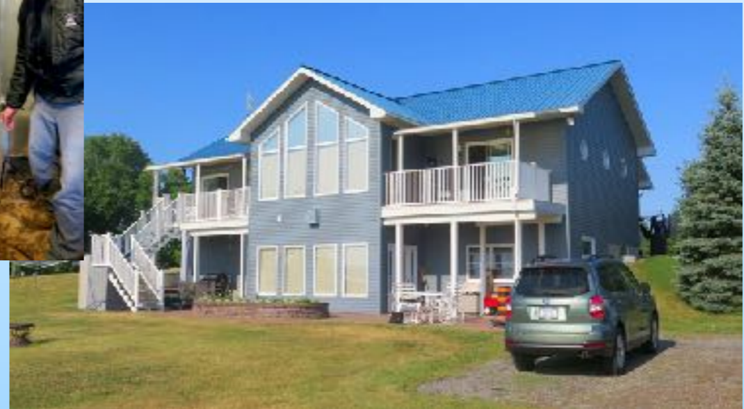
MORRISBURG, ONTARIO, ONE OF HUNDREDS OF GEOHERMAL RETROFITS (PHOTO OGA)
