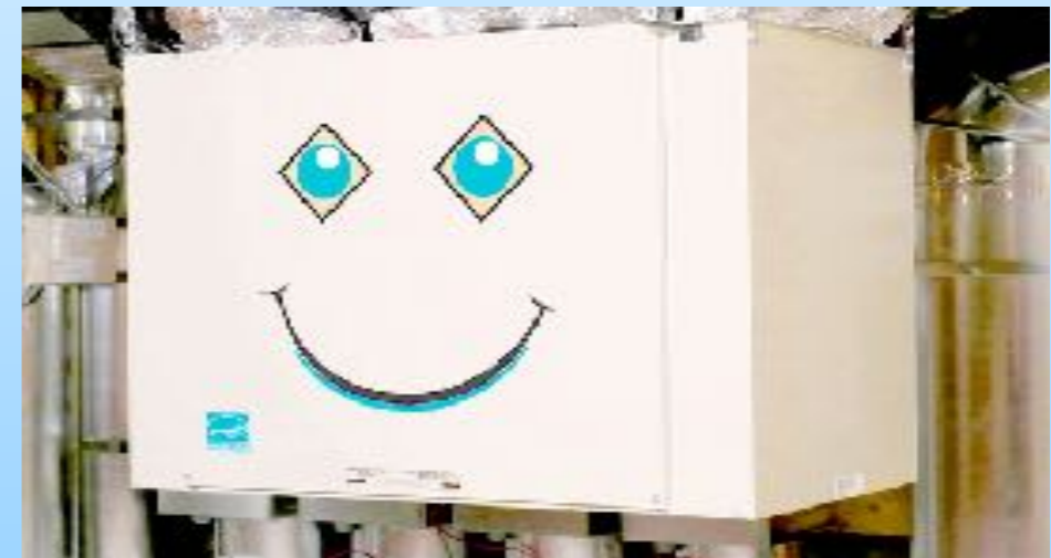
Heat Recovery Ventilator (HRV)
