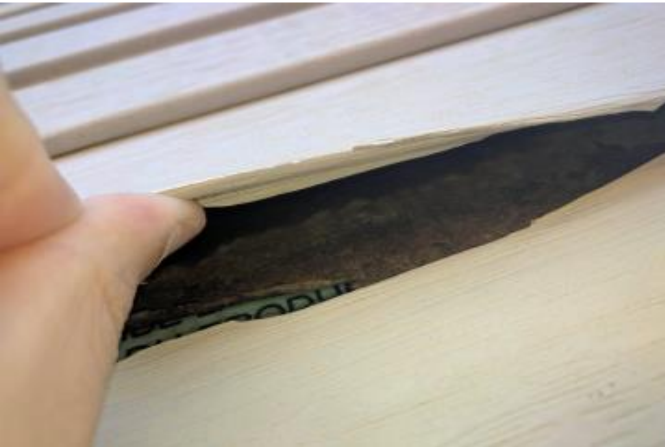
Vinyl Deteriorating
