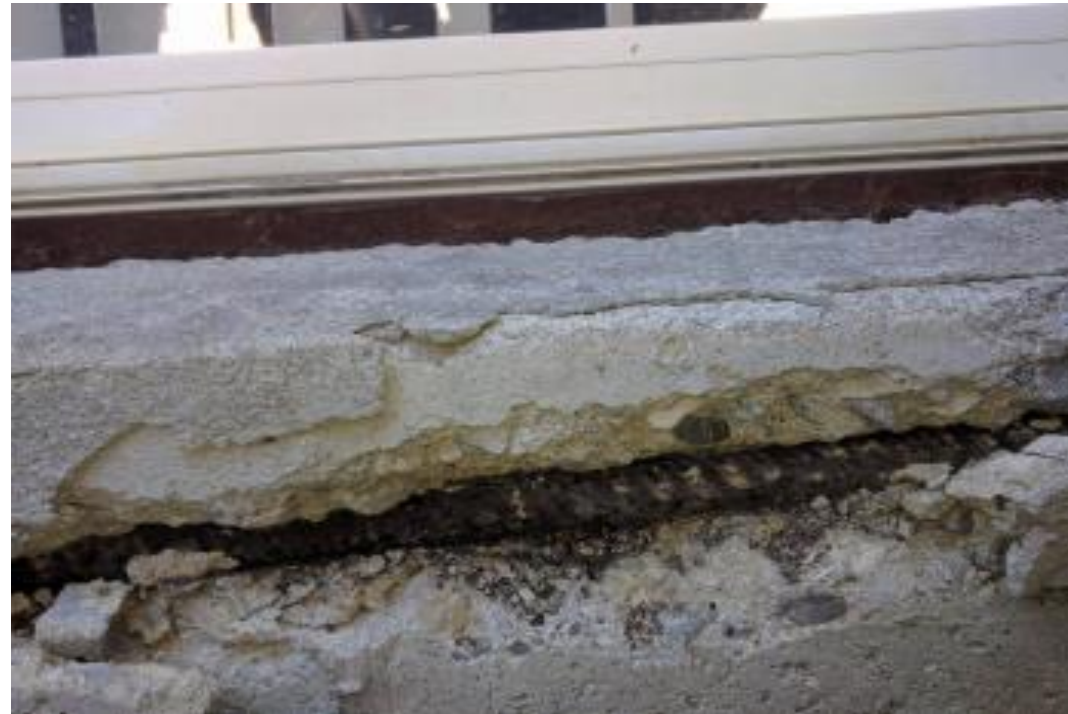
Exposed Rebar
