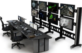
Network operation center
