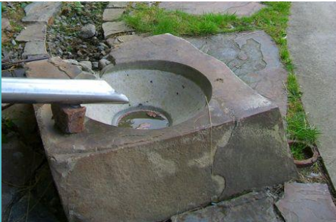
Downspout disconnect to perforated cistern
