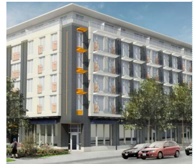
Highly energy efficient wood-frame residential building under construction in Vancouver (Part 3, Step 4)
