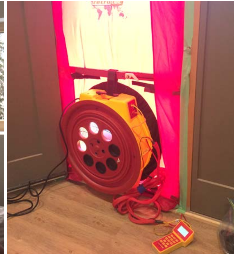
Right: Blower door testing during a builders' workshop held in Invermere; the home is expected to exceed EnerGuide84 (equivalent to Part 9, Step 3).
