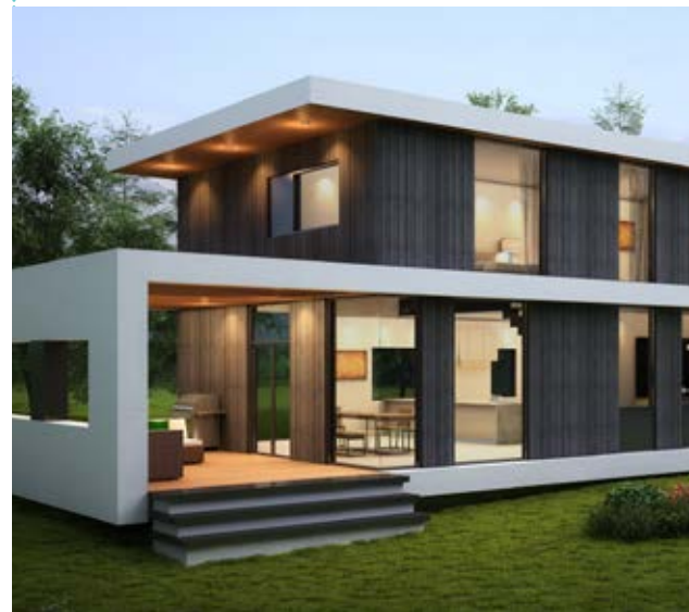
Highly energy-efficient home currently under construction in Kelowna, by Marken Design + Consulting (Part 9, Step 5)
