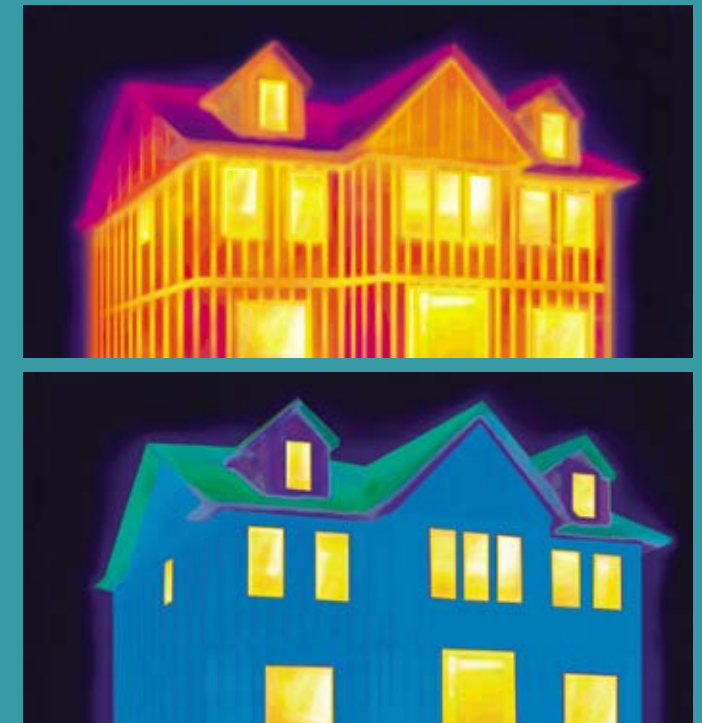
Figure 6: Example thermal images of a building demonstrating thermal bridges. Areas that are red and yellow show a lot of heat escaping through the building envelope. Blue and green areas show much less heat is escaping. Photo credit: Dow Chemical Company.
