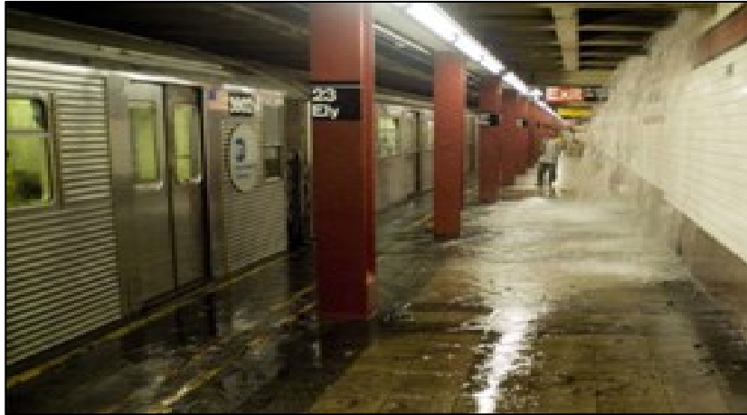
NYC subway flooding after a 2007 storm.
