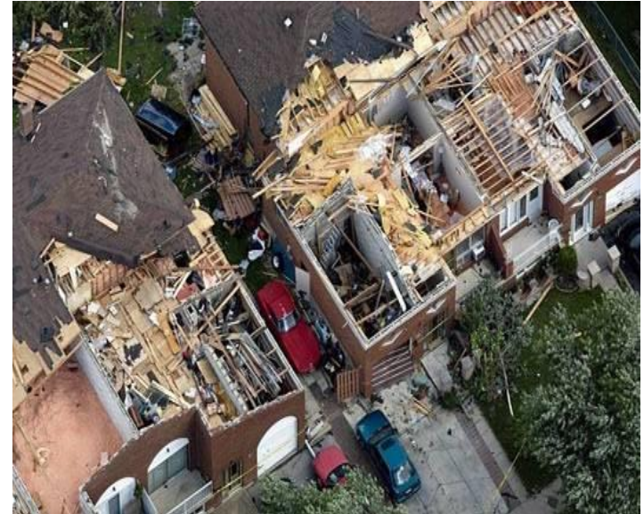
Tornado damage in Vaughan, 2009
