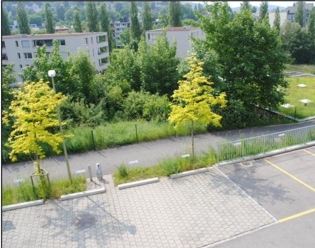
Green technologies Eg. Permeable pavement
