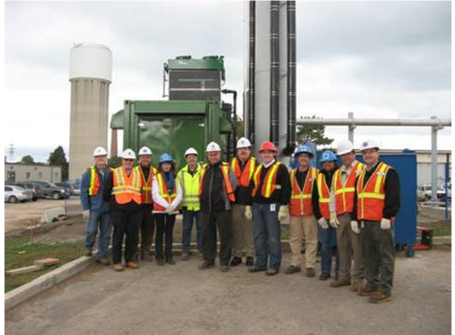
BioGas Purification Unit
