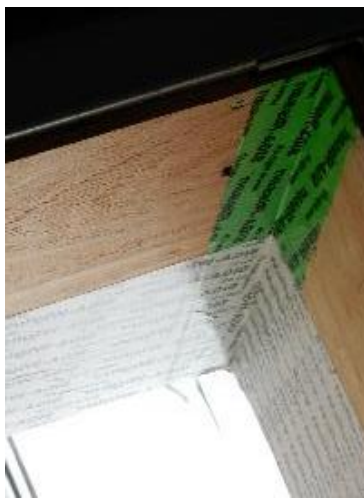
Vapour control: Lap to primary vapour control layer
