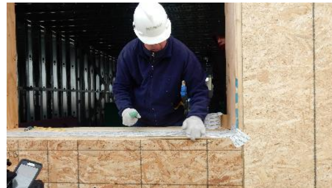
Airtightness at window opening
