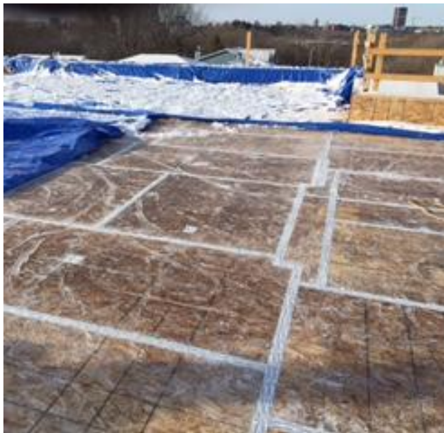
All service penetrations are meticulously taped for state of the art airtightness
