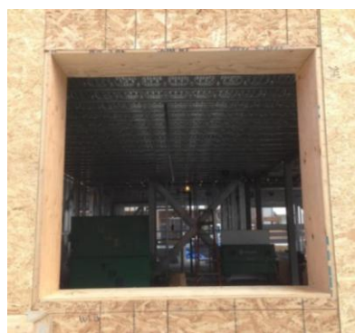
Plywood box install
