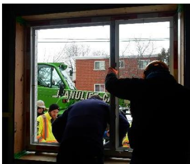
Window is set and screwed in place
