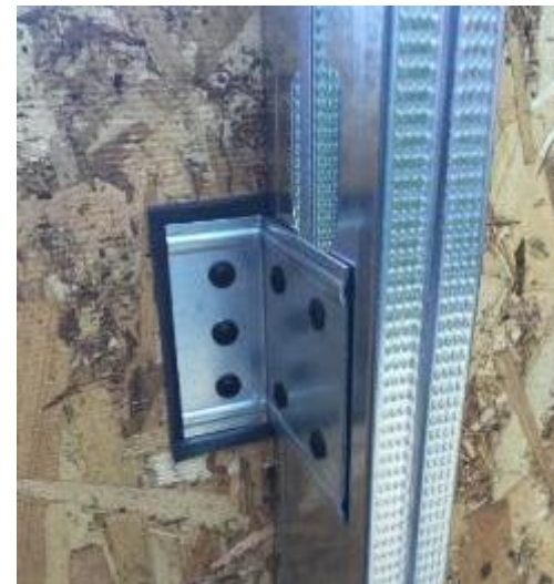
air tight installation at the Steel brackets with Siga Nail Seal Tape
