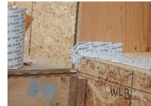
Lap to primary airtightness layer
